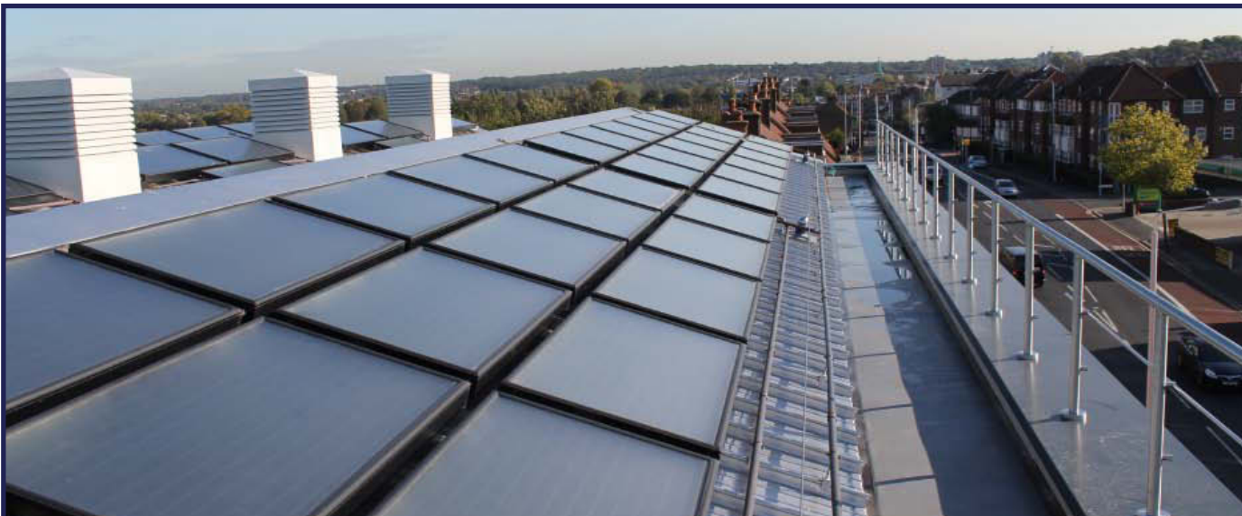
PV-T panels in-situ on Walthamstow Fire Station provide electricity and heating for the station
